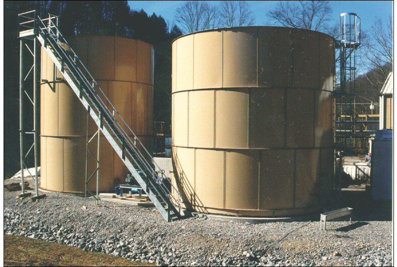
Hybrid and SBR under construction
